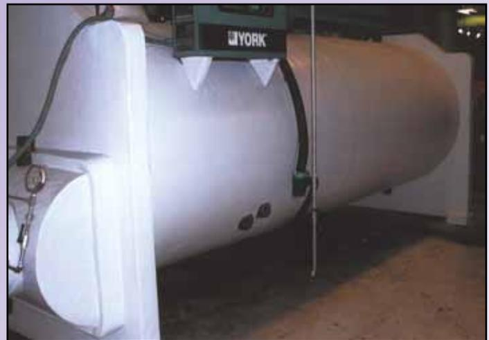
The above application shows a chiller that was insulated in a mechanical room with rubber insulation and covered with VentureClad® 1577CW-WM. VentureClad jacketing offers the following advantages for insulation jacketing applications:
