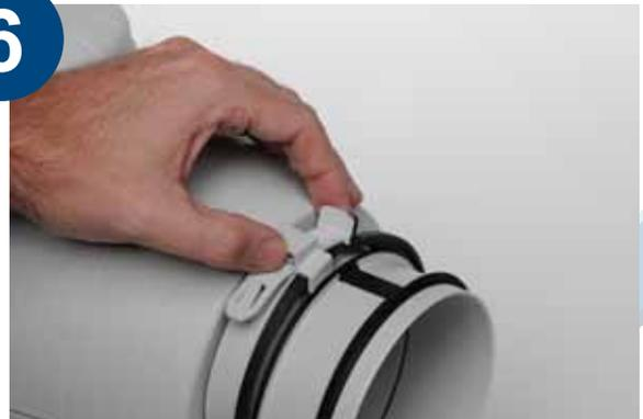
Re-mount fan body by tightening the clamps.
