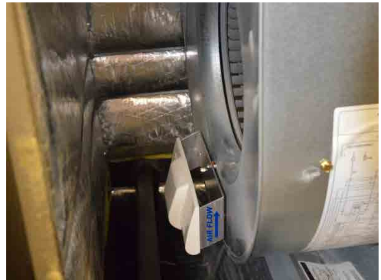
QUAD-DM™ mounted to blower housing
