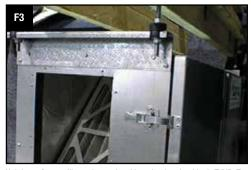
Unit hung from ceiling using optional hanging bracket kit, 45EVHB. To install hanging bracket, identify the corners of unit you wish to hang it from. Remove existing screws from unit pan. Attach hanging bracket to unit using screws provided with the hanging bracket.
