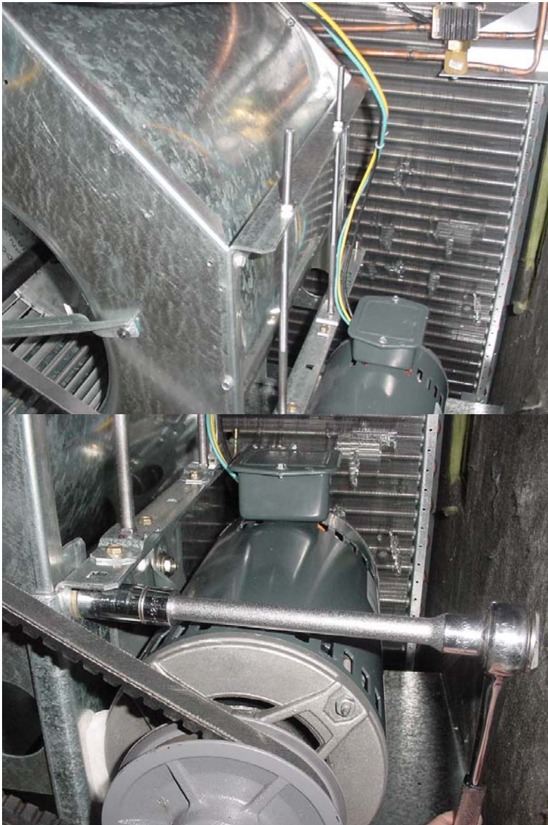
Figure 8 – Belt Tension Adjustment
