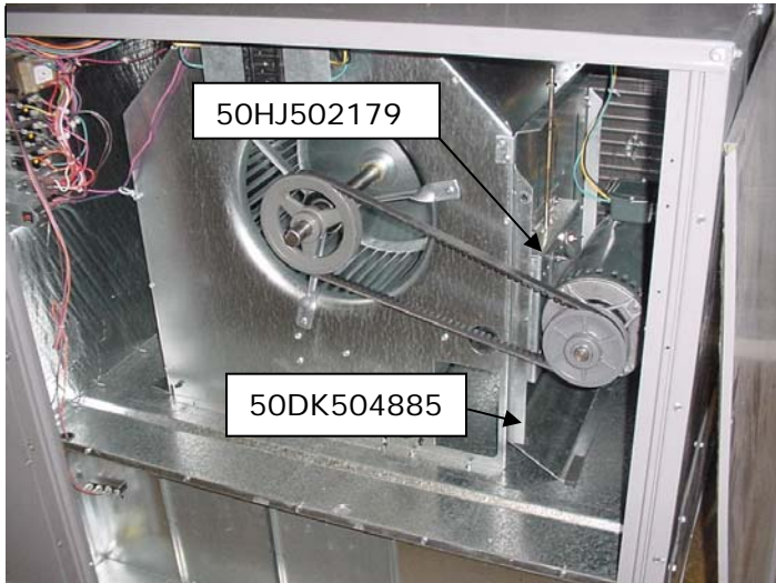
Figure 1 - Existing motor mount hardware.
