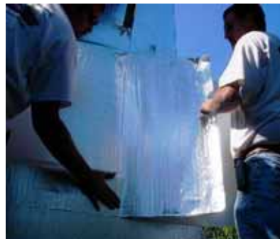
Pull release film from behind membrane and continue to press into place.
