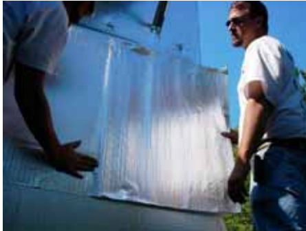
Remove release paper, align membrane and press to stick.
