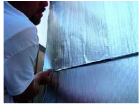
Position FlexClad-400 into place.
