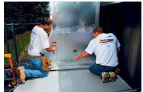
Roll entire surface firmly with a hand roller to ensure good adhesion.
