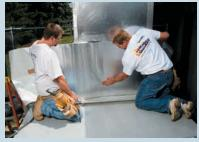
After measuring and cutting the section to the proper size, align and gently press FlexClad into place; reposition if necessary.
