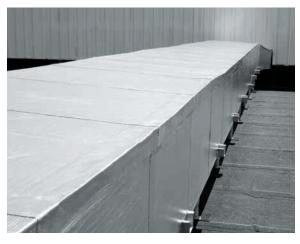
Properly applied, FlexClad creates a protective barrier against inclement weather, and the UV-resistant aluminum top surface reflects sunlight to reduce interior temperatures and energy costs. Durable, protective and self-sealing around punctures, it conforms to and effectively seals around external support brackets.
