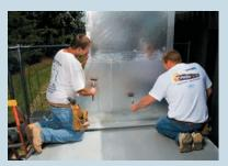
Complete the installation by applying firm pressure to the entire surface with a hand roller.
