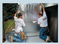
Cut the next section to size. Overlap the previous section by at least 3" in order to create a secure, water-resistant seal.
