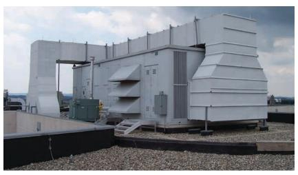
The aluminum top surface is an extremely durable laminated film that is both highly tear and puncture-resistant. FlexClad is also available in different color choices to blend your system to the surrounding structure.
