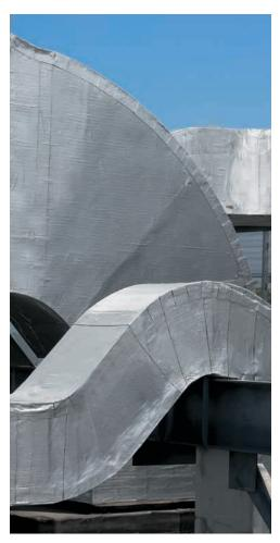
Count on the highly aggressive rubberized asphalt adhesive on FlexClad to securely stick to rigid board insulation protecting it from weather damage and deterioration. Note: On installations involving curved shapes and edges, metal angle should be used to prevent corners of the insulation material from deforming and to give a neat, finished look.
