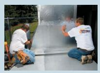
When in final position, firmly hand seal to the surface and fold over all edges as shown.
