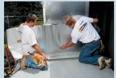
*After measuring and cutting the section to the proper size, align and gently press FlexClad into place; reposition if necessary.*
