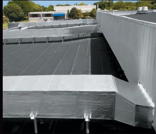
*For straight, long length duct systems, FlexClad makes for a clean, uncluttered appearance. Quickly and easily installed, it replaces expensive and cumbersome metal jacketing commonly used to protect insulated ductwork.*
