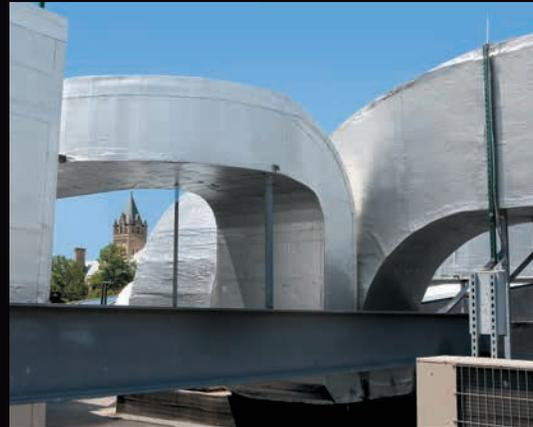
*Potentially difficult installations that include sweeping curved corners and odd shapes are made easy with FlexClad, and its excellent elongation characteristics accommodate structural movement.*
