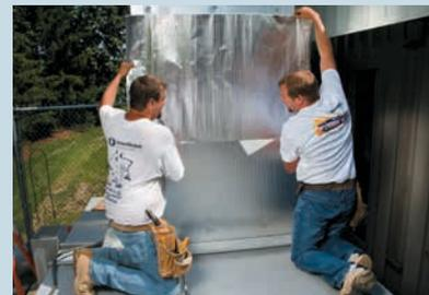
*Cut the next section to size. Overlap the previous section by at least 3" in order to create a secure, water-resistant seal.*
