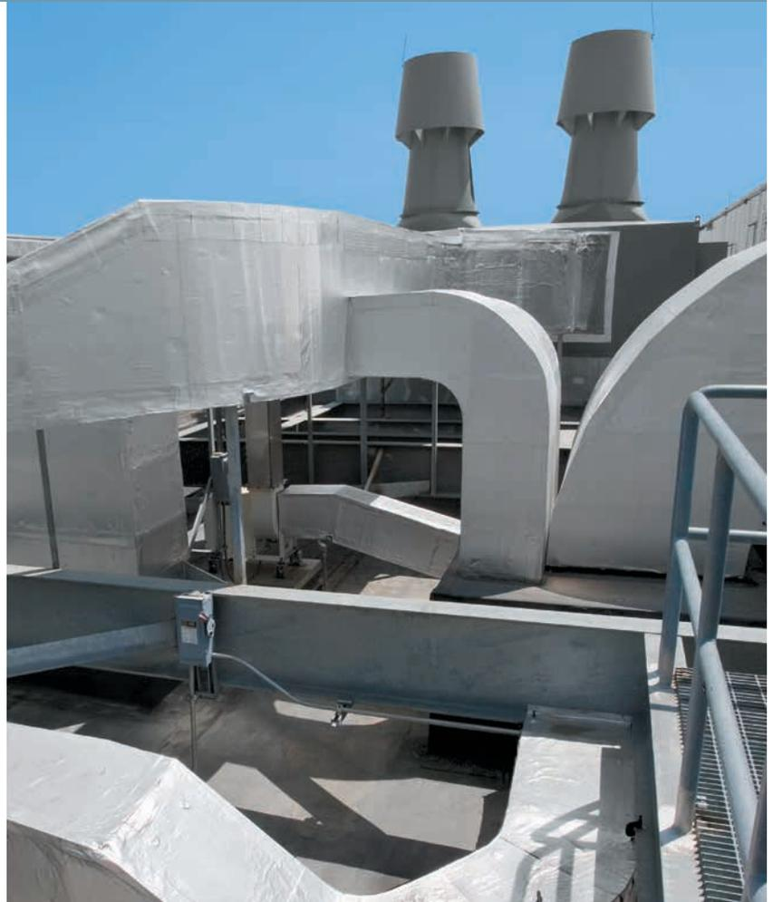
*FlexClad can be applied to virtually any shape or configuration. It completely protects the ductwork from infiltration of outside moisture and harmful sunlight, and is warranted by MFM for 10 years.*
