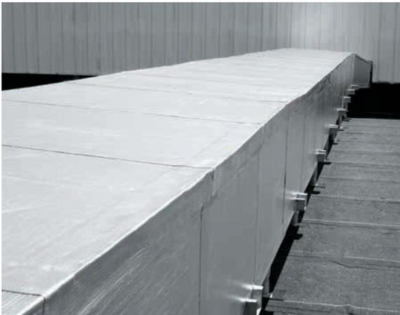
*Properly applied, FlexClad creates a protective barrier against inclement weather, and the UV-resistant aluminum top surface reflects sunlight to reduce interior temperatures and energy costs. Durable, protective and self-sealing around punctures, it conforms to and effectively seals around external support brackets.*
