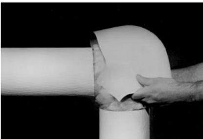
4. Insert two stainless steel serrated tacks approximately ¼" (6 mm) from one of the lap edges of the fitting cover. Then snap the cover in place over the fiber glass insulation.
