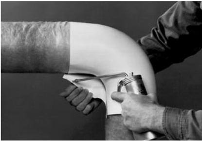
2. Using a standard applicator gun or squeeze bottle, apply a bead of Perma-Weld adhesive along the throat overlap of the fitting cover. Snap the fitting cover into place and secure with elastic cord or PVC tape. Always feather the adhesive along the seam.
