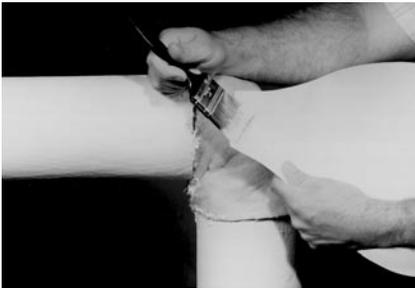
4. Apply the mastic along the inside of the fitting cover throat overlap seam. Pressure-sensitive Z-Tape or serrated tacks may also be used.
