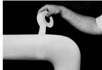
6. Apply Z-Tape over the circumferential joints. The tape should extend over the adjacent pipe insulation and overlap itself by at least 2" (51 mm) on the downward side of the lap. The tape provides securement, an attractive appearance, and completes the vapor seal.
