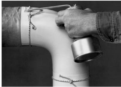
3. After the fitting cover has cured at least 10 minutes, run a bead of adhesive along its circumferential edge. Overlap the fitting cover (by approximately 1" [25 mm]) with a section of Zeston PVC jacketing and secure the circumferential joint with an elastic cord. The cord may be removed after approximately 10 minutes.
