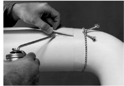
4. Overlap the jacketing on itself (approximately 1½" to 2" [38 mm to 51 mm]) and apply a bead of adhesive along the entire length of the longitudinal lap. Place elastic cords or PVC tape around the jacketing.
