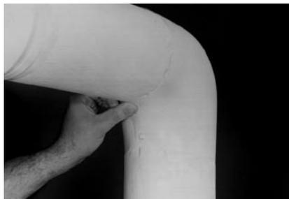
5. After the fitting cover is in position, push the tacks into the overlapping throat seam. No further fastening is required.
