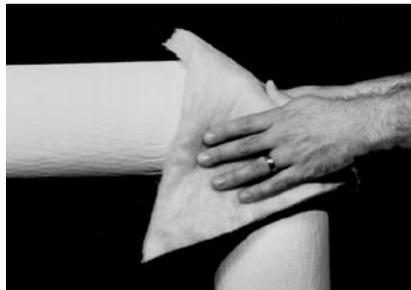
2. Place the pre-cut fiber glass insert around the fitting, positioning the points of the insert on the inside radius of the elbow. For applications with temperatures below 45°F (7°C) or above 250°F (121°C), additional layers of insulation may be required.\* In such cases, the first layer is secured by wrapping with fiber glass yarn.
