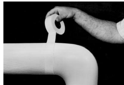
6. As an option, apply color-matched, pressure-sensitive Z-Tape to the butt joints for a more attractive appearance.
