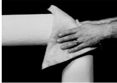
2. Position, tuck, and fold the fiber glass insulation insert as described below in steps 2 and 3 for hot systems.
