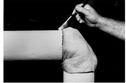
3. Apply a vapor barrier mastic around the edges of the adjoining pipe insulation.
