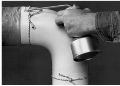
3. After the fitting cover has cured at least 10 minutes, run a bead of adhesive along its circumferential edge. Overlap the fitting cover (by approximately 1" [25 mm]) with a section of Zeston PVC jacketing and secure the circumferential joint with an elastic cord. The cord may be removed after approximately 10 minutes.
