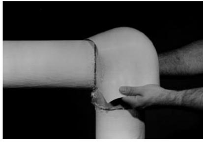
5. Place the fitting cover over the insulation, lapping the mastic-covered edge over the other side of the throat seam.
