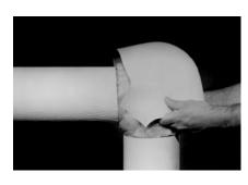
4. Insert two stainless steel serrated tacks approximately ¼" (6 mm) from one of the lap edges of the fitting cover. Then snap the cover in place over the fiber glass insulation.
