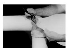
Apply the mastic along the inside of the fitting cover throat overlap seam.
