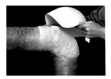
1. Position the Zeston PVC fitting cover over the insulated fitting.
