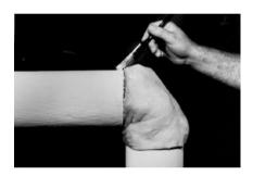
3. Apply a vapor barrier mastic around the edges of the adjoining pipe insulation.
