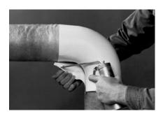
Using a standard applicator gun or squeeze bottle, apply a bead of Perma-Weld adhesive along the throat overlap of the fitting cover. Snap the fitting cover into place and secure with elastic cord or PVC tape. Always feather the adhesive along the seam.
