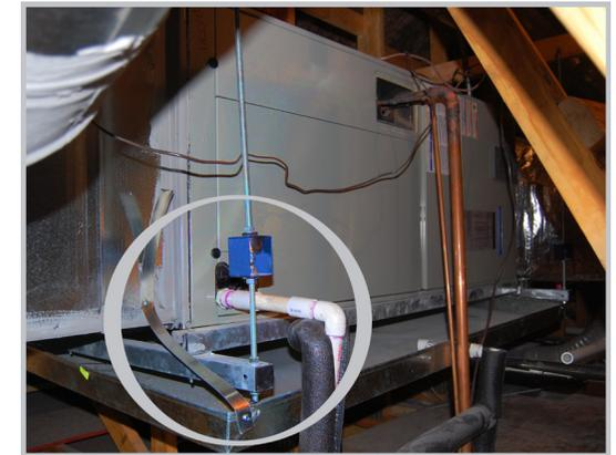
For commercial installations, use threaded rod for added support!
