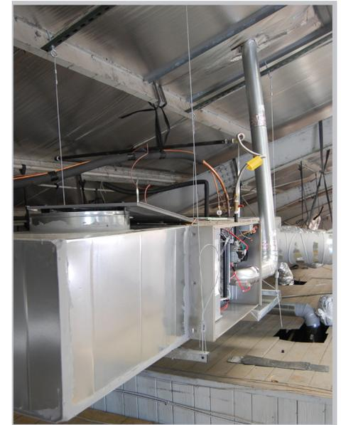
The use of cable & cable locks allow for the bolt to be set in a variety of places with a maximum cable angle of 45°
