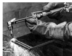
Figure 19. Steel Flame Cutting
