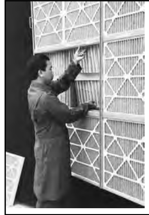
Installing filters and prefilters
