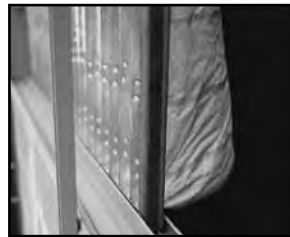
Filters with poly-foam side gasket prevent leaking between adjacent filters
