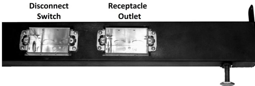
**Figure 6 – Junction Boxes Installed**
