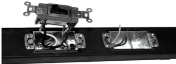
**Figure 12 – Install wiring for Receptacle**
