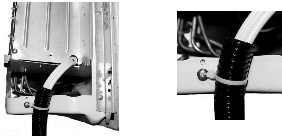
Figure 14 – Install Conduit Strain Relief
