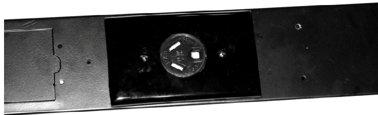
Figure 10 – Install Receptacle Cover
