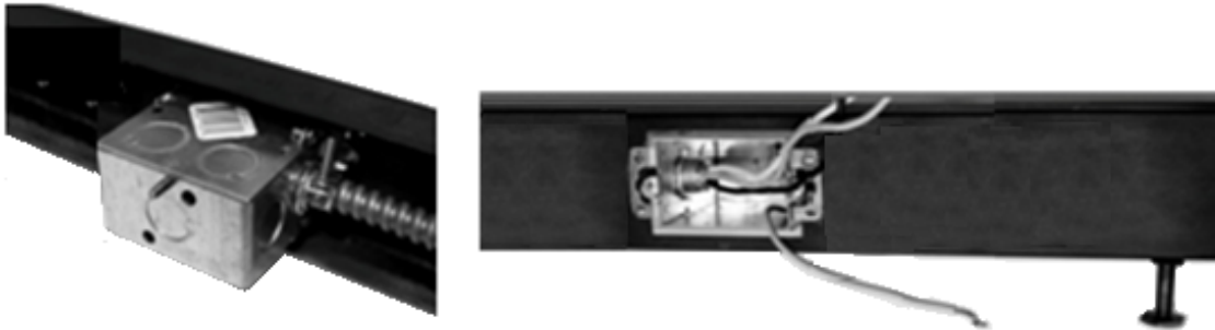
Figure 7 – Attach Conduit to Junction Box
