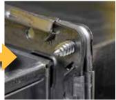
The teardrop shaped cut out of the corner with the proprietary bolt pull the connection together and lock it in place without the use of a nut, using a convenient cordless impact driver.
