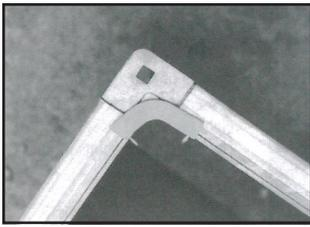
14. On the mating WDCI frame apply 440 gasket only to the corners as in photo (approximately 3" per corner). The same 3 point application requirements apply as in photo 12.
