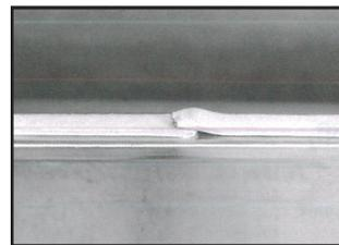
13. Apply 440 gasket completely around WDCI frame to the beginning point. Where the gasket meets overlay about  $\frac{3}{8}$ ".
