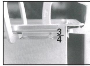
10. It is essential that the frame angle is fastened to the duct within  $\frac{3}{4}$ " of the end of the angle at each corner.
