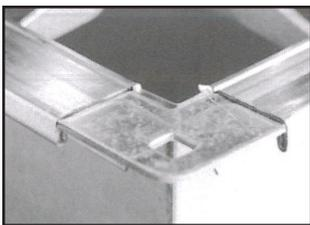
8. The duct must be seated all the way into the WDCI angle in order to penetrate the integral mastic sealant and avoid leakage.
