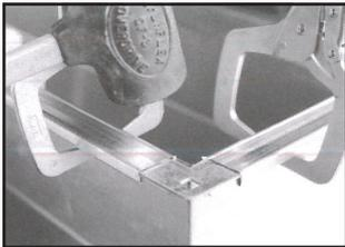
7. Use a mallet to seat the frame onto the duct. *Establish metal to metal contact along the length of the angle.*
