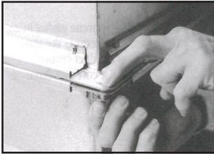
16. Insert  $\frac{3}{8}$ " x 1" nut and bolt for WDCI J Connection System.
