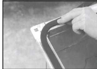
3. Position Neoprene gasket in an arc so that it covers the three points in the duct corner. Gasket must cover all three points.
