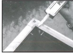
1. Apply a liberal amount of PROseal sealant in each of the eight corners. The sealant must cover the three points in the duct corner.
