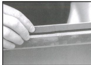
4. Apply Neoprene gasket completely around WDCI frame to the beginning point. Butt the two ends of the gasket up against each other. Do not overlap the two ends.
