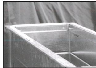
11. Start approximately in the middle of one side, place a single strip of gasket tape completely around the inside edge of the angle frame. At the corners, the gasket must cover the exposed edge of the duct section and the gap between the duct wall and the WDCI corners.
