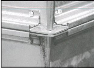
15. Carefully align mating frames before they touch. Ductmate 440 adheres on contact. A drift pin can be used to correct any misalignment.
