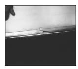
Apply 440 gasket completely around Ductmate frame to the beginning point. Where gasket meets overlay about 3/8".
