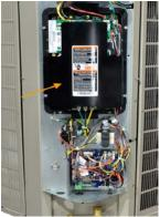
3. Use a 5/16" nut driver to disconnect the (3) power wires going into the inverter (from the contactor). Remove the ground wire from the ground terminal of the fuse board.
