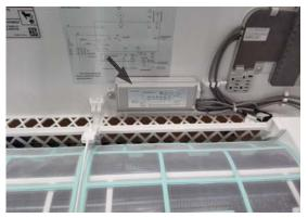
**Fig. 22** – Multi–Function Board 2. Disassemble the Multi–Function Board.
